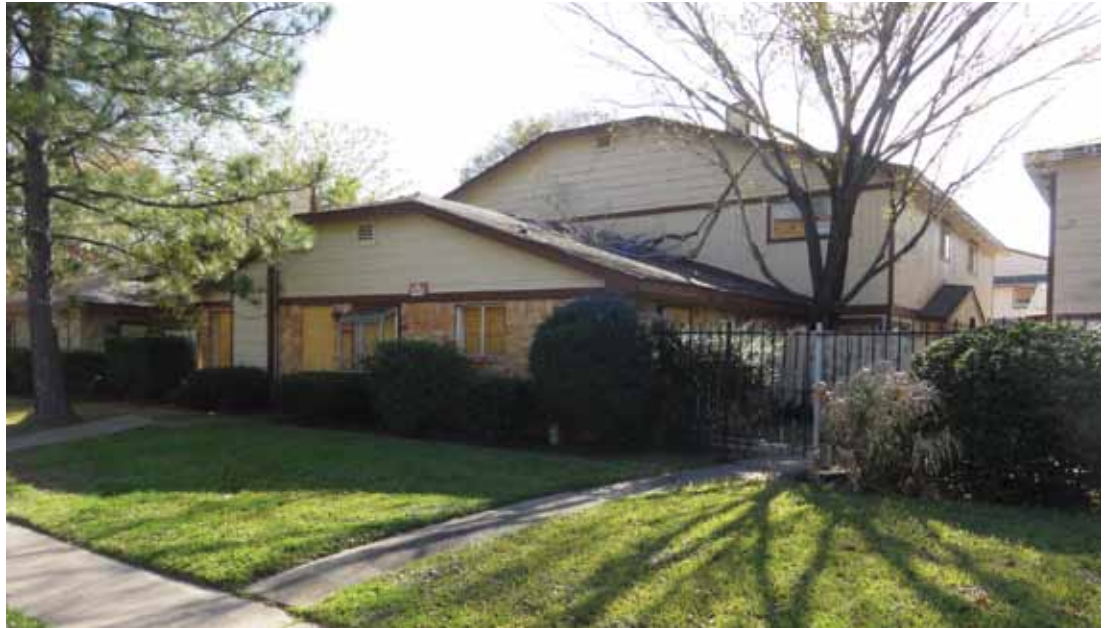
Vacant units for lease on De Soto Street in Near Northwest Houston.
