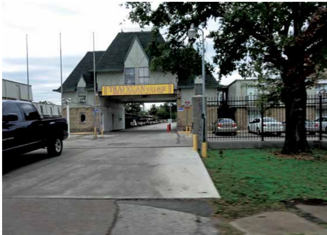
The Thai Xuan Village condominiums along Broadway have struggled to fund needed maintenance.
